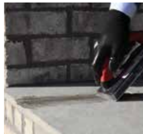
PIC 1. Fill joint with grout.
