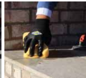
PIC 2. Remove excess grout with clean water.
