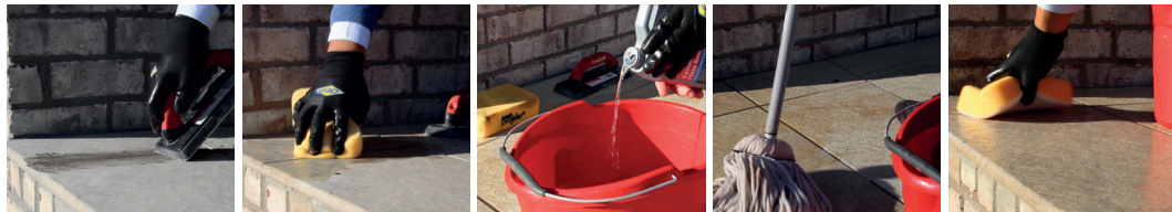
PIC 1. Fill joint with grout.
