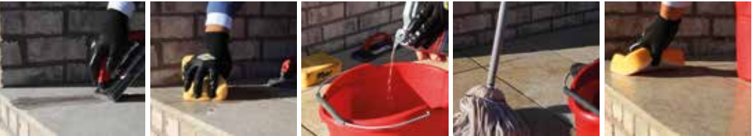
PIC 1. Fill joint with grout.
