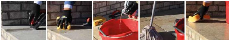
PIC 1. Fill joint with grout.
